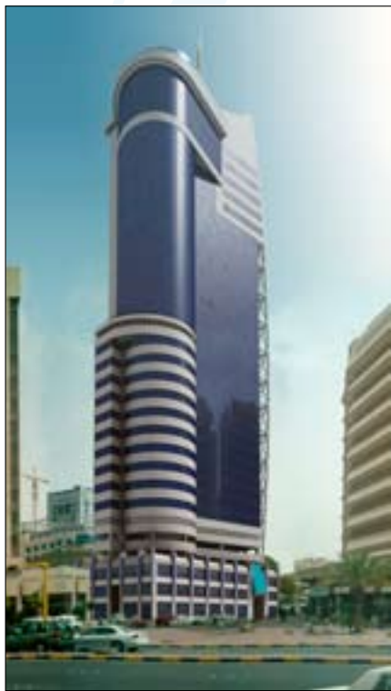
Österr. Know-How in Kuwait City Al Jawhara Tower
